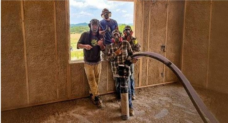
around a job site. Hempcrete does not shrink, maintains a steady temperature, and can also increase in strength over time. In addition, hemp and lime based biocomposite
